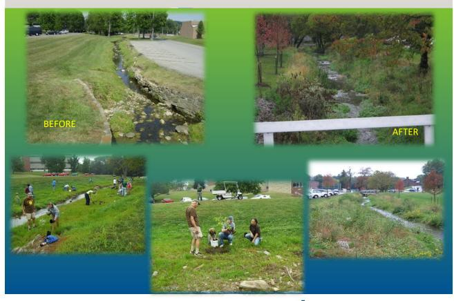
The McClure Run Watershed Restoration Project consisted of restoring and enhancing 1,685 linear feet of McClure Run using Natural Stream Channel Design techniques to promote a stable stream corridor and improve aquatic health. Westminster College received a PADEP Growing Greener grant to complete the stream restoration which flows through the college's campus.
