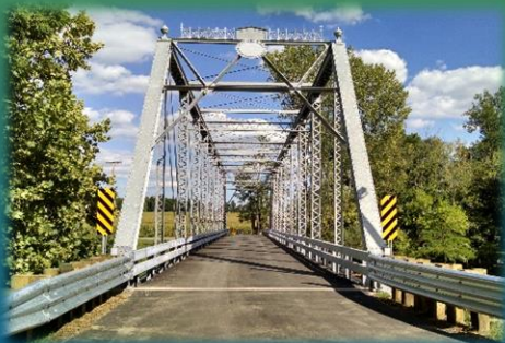
Rehabilitated Bridge West View
