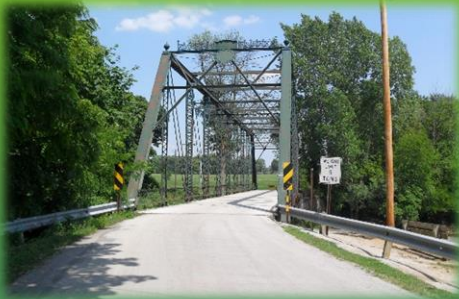
Former Bridge West View
